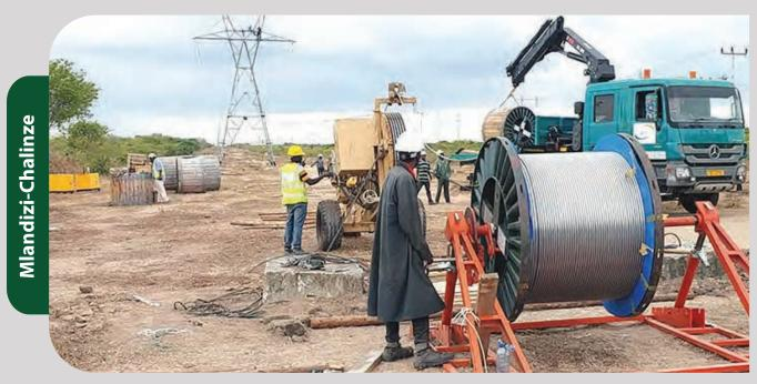
Preperation and rolling of conductors during the replacement of old ones.
